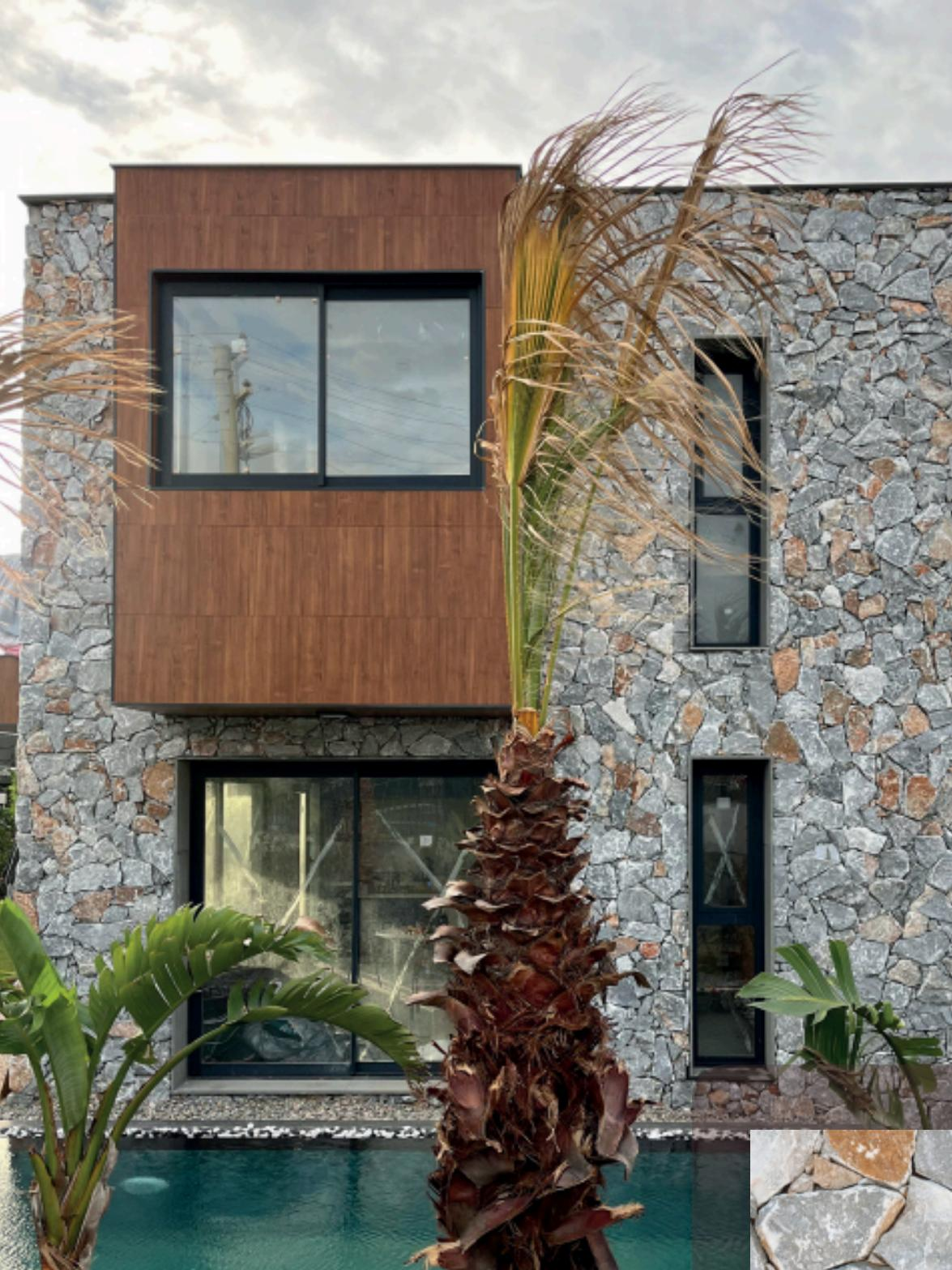
The Grey Nature Rockshell model is created by crushing the rubble from the grey marble quarry and thinning it down to 2 cm, preserving its surface form.
