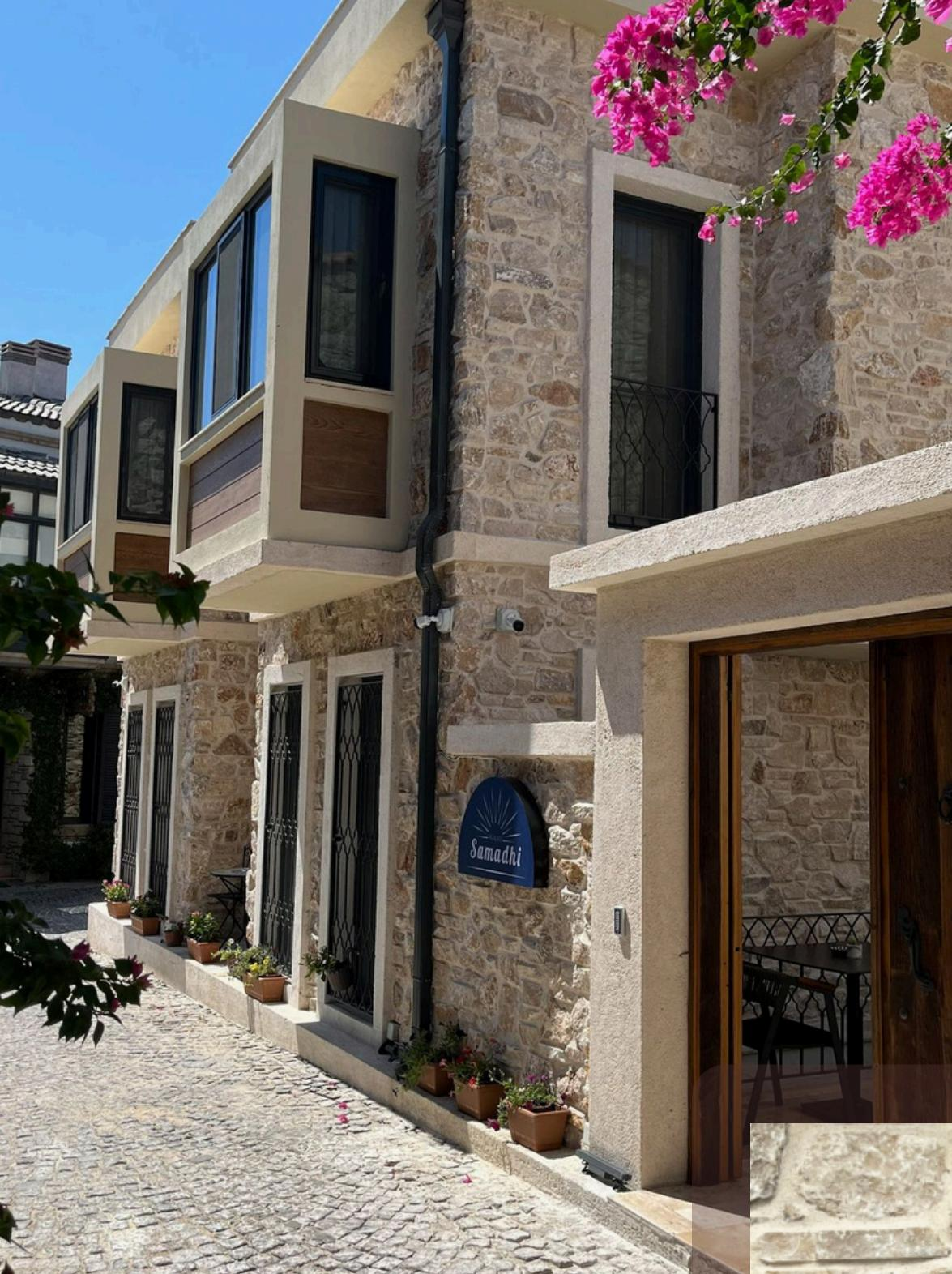
The Scabas Mix Rockshell model is created by crushing the rubble from the Scabas travertine quarry and thinning it to a thickness of 2cm, then mixing natural stones with dimension stones on a horizontal plane.
