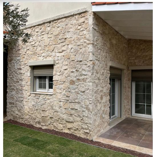
The Mixed Rockshell model is created by mixing unsized, plump stones with stones that are thin and sized in horizontal planes.
