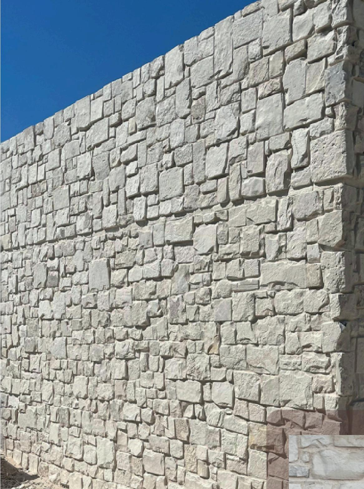
The Limra Mix Rockshell model is the result of mixing natural stones with dimension stones on a horizontal plane after crushing the rubble from the Ören limestone quarry and thinning it to a thickness of 2 cm.
