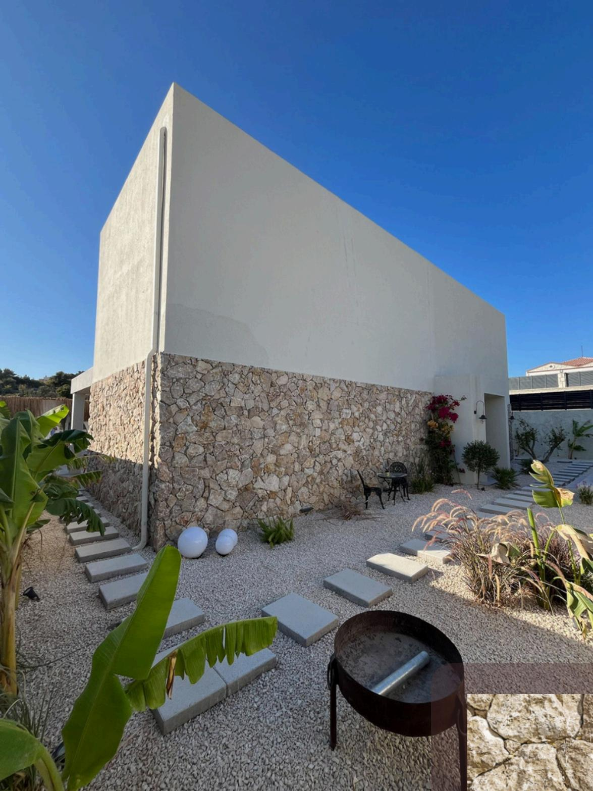
The Noche Nature Rockshell model is created by crushing the rubble from the noche travertine quarry and thinning it down to 2cm, preserving its surface form.
